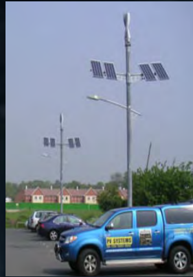
PV cells for Car park lighting
