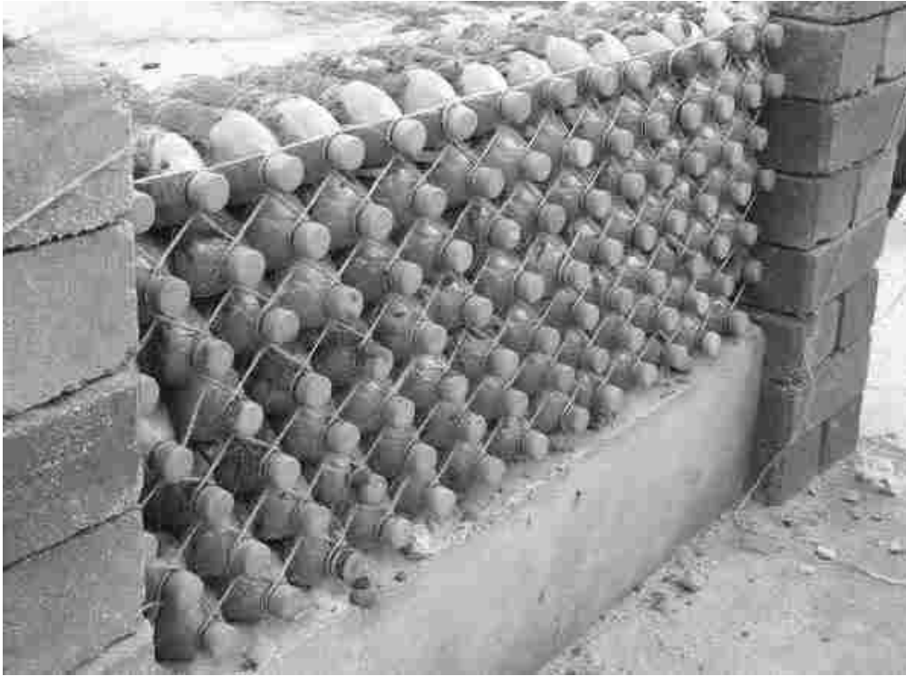
Figure 4.6: The experimental bottle wall constructed in Chamazi. The lower part of it, which was completed one week earlier, was covered with cement plastering. Photo by: Qidi Jiang, 2013
