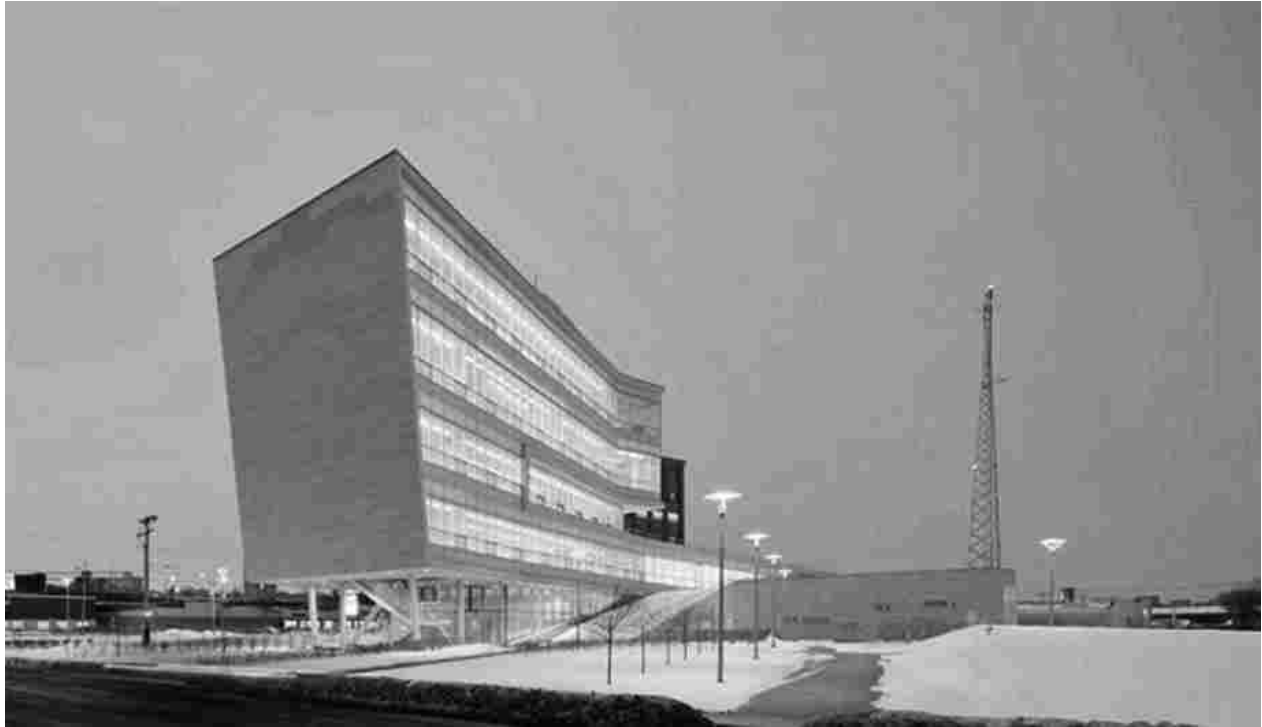
Figure 4.9: The Syracuse Center of Excellence (SyracuseCoE), photo by: Ivan Baan . Housing 5,110 square metres of lab and classroom space, the Center of Excellence provides state-of-the-art lab space for pioneering research. The structure's green innovations provide these amenities with low environmental impact. To cut electricity use, a narrow building profile maximizes the penetration of daylight; windows employ glazing and automated microblinds to reduce glare; and lighting is activated by sensors in response to need. Rainwater reclamation supplies all toilets and the irrigation of the green roof. Radiant heating and cooling, natural ventilation and a geothermal borefield of 49 wells reduce the climate control's demand on the grid. Rapidly renewable materials were used wherever possible, including in the insulation. Even its site – formerly a brownfield contaminated with chromium, oil, and asbestos – has been renewed to represent the revitalization of an entire neighbourhood, a dash of green in an area once in danger of falling off the map. ( Dick-Agnew (2011) )
